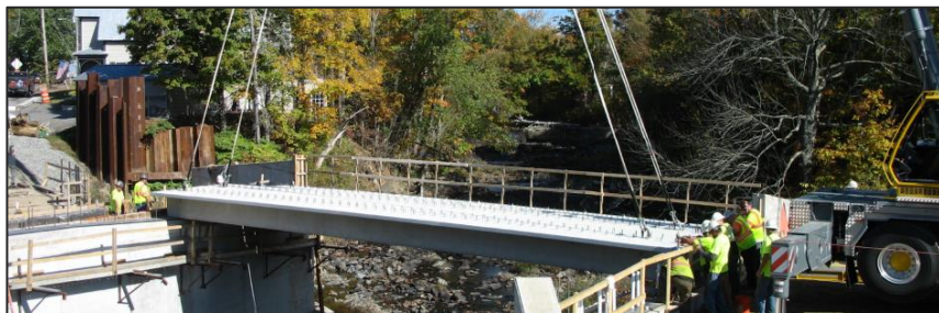
Installation of girders/deck
