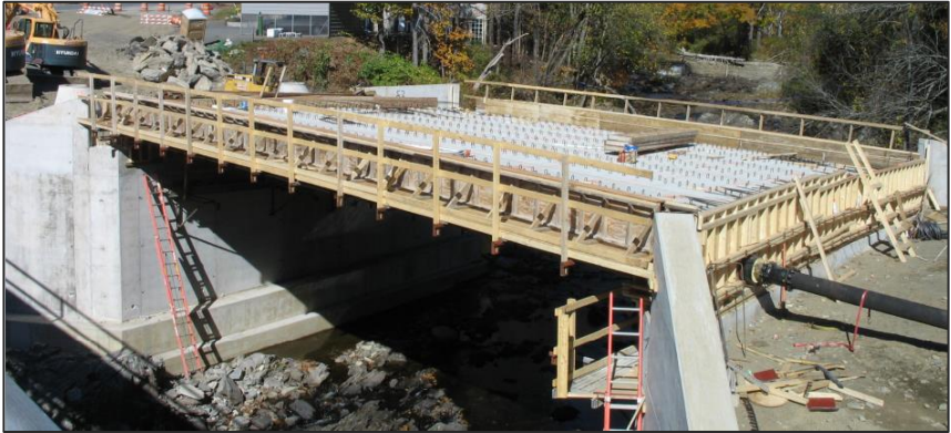
Framing and prep for concrete slab base
