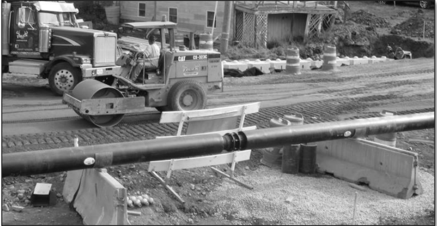
Water Main pipe reinstallation for under new bridge.
