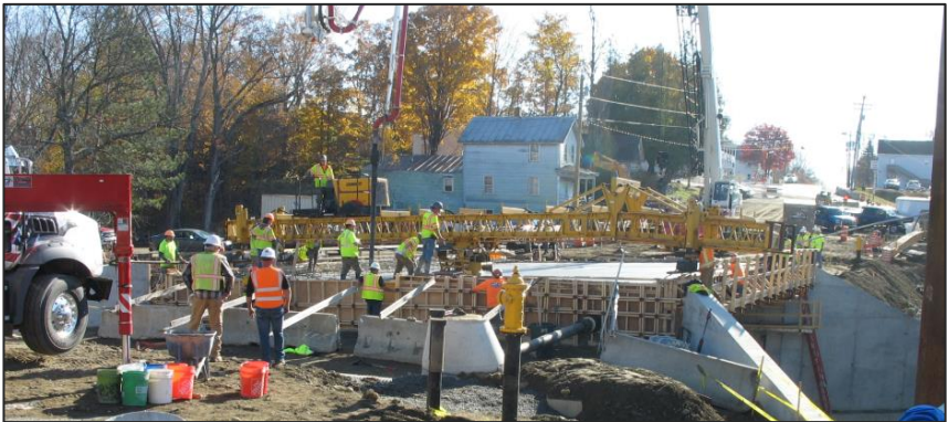
Concrete slab installation and finish
