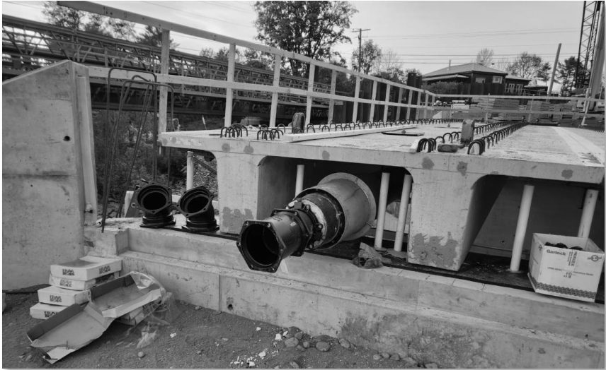
New water main positioned under the west side of the new bridge
