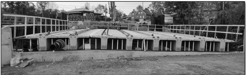
New water main positioned under the west side of the new bridge
